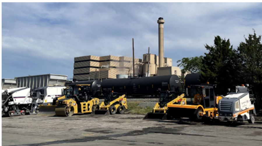
Figure 4: ReWorld (formerly Covanta) and railway to the south of the subject property
