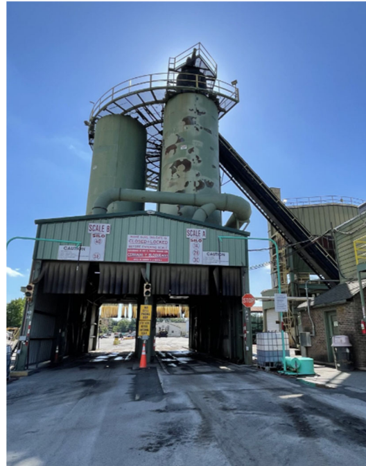
Figure 7: Asphalt loading facility
