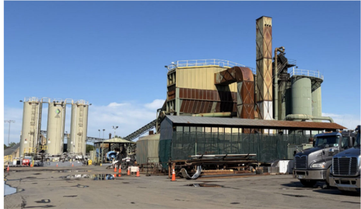
Figure 1: Virginia Paving asphalt production facility
