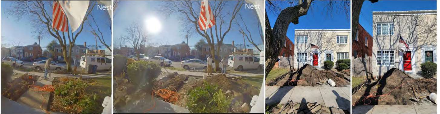
Day 2 Feb 9: Sidewalk and concrete step demolition, raised planter beds footing excavation
