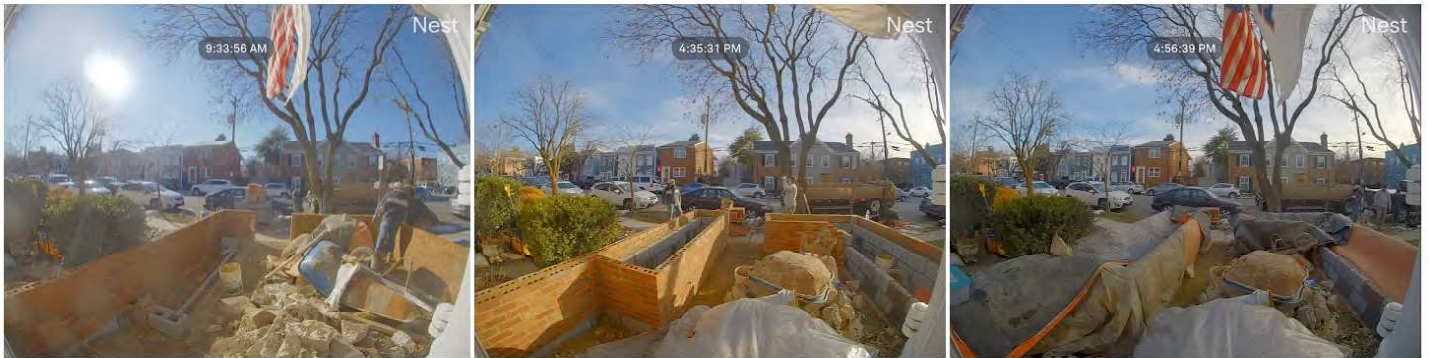
Day 6 Feb 22: Brick walls installation continues with CMU backing. Due to freezing temperatures, a torch is being used to heat the bricks and grout for installation.
