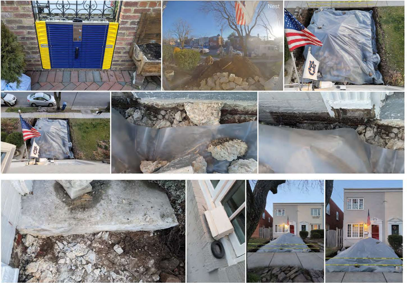
Day 3 Feb 10: Continued excavation, footing rebar install, footing concrete poured. Site was covered for concrete to cure through the rain and freezing temperatures.
