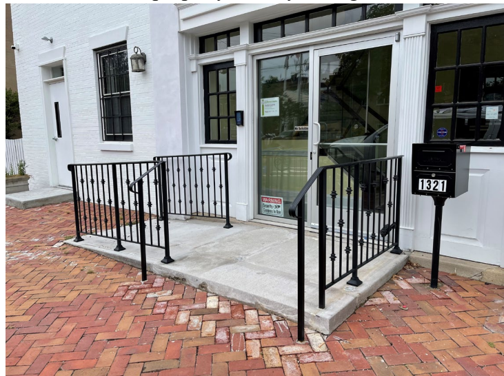
Figure 2: New ADA ramp at the entrance of the day care
