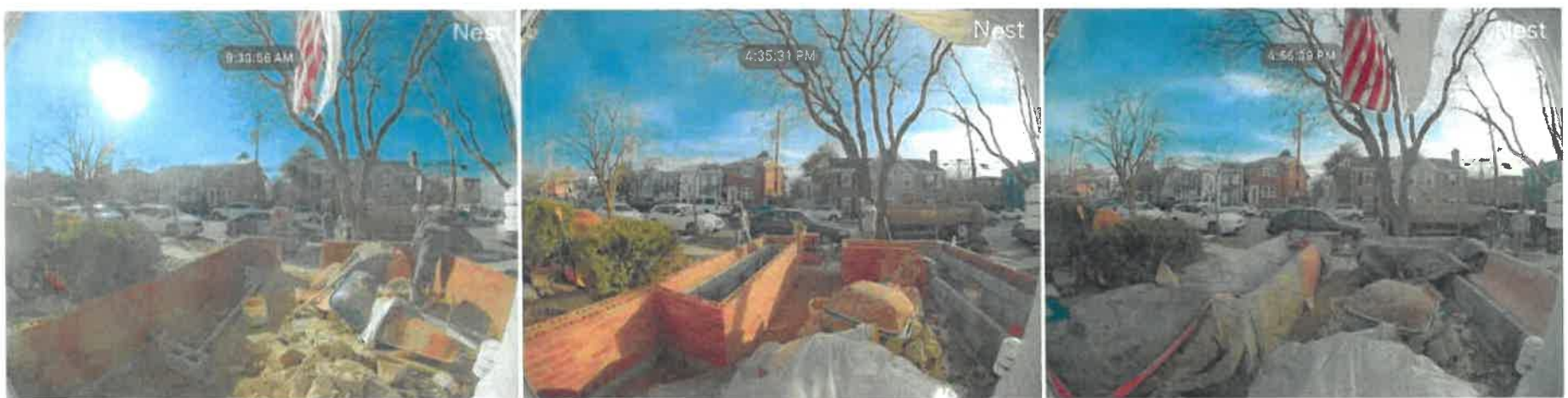
Day 6 Feb 22: Brick walls installation continues with CMU backing. Due to freezing temperatures, a torch is being used to heat the bricks and grout for installation.
