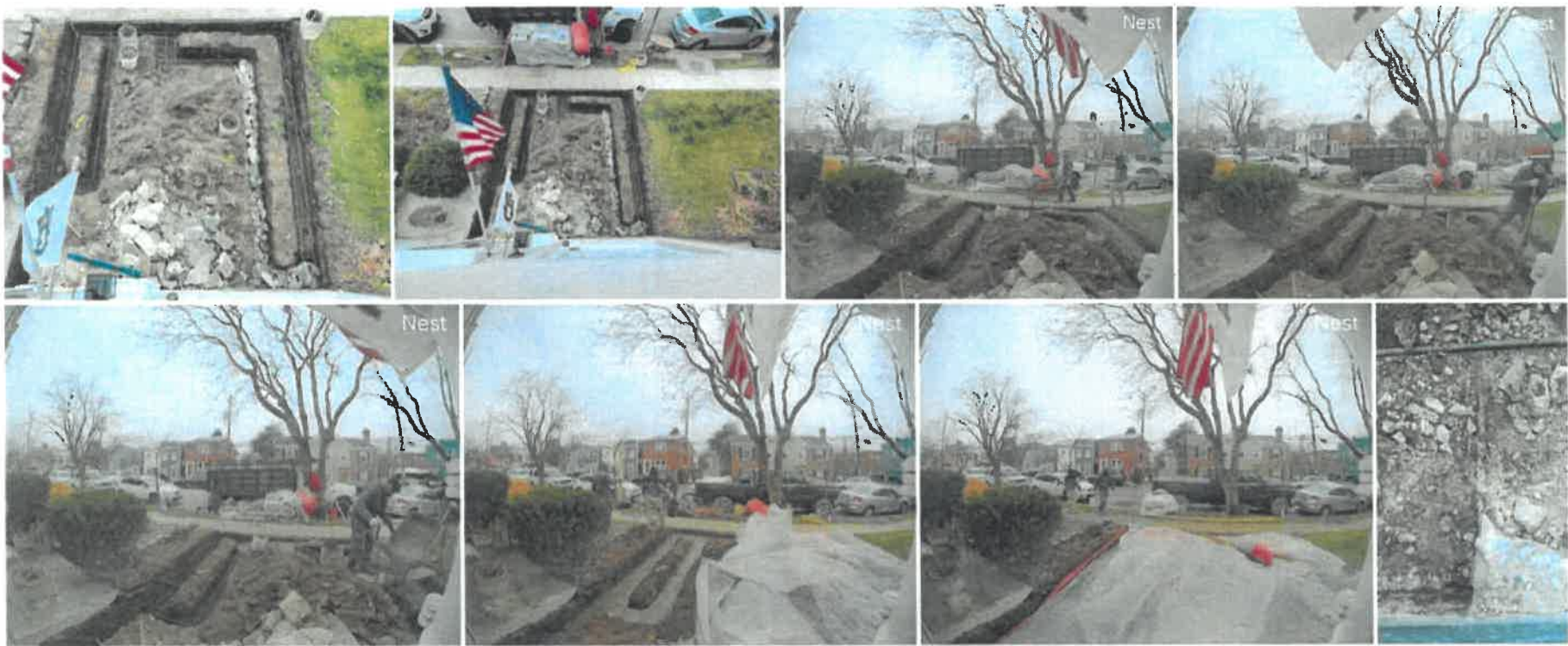
Day 3-Feb 10: Continued excavation, footing rebar install, footing concrete poured. Site was covered for concrete to cure through the rain and freezing temperatures.
