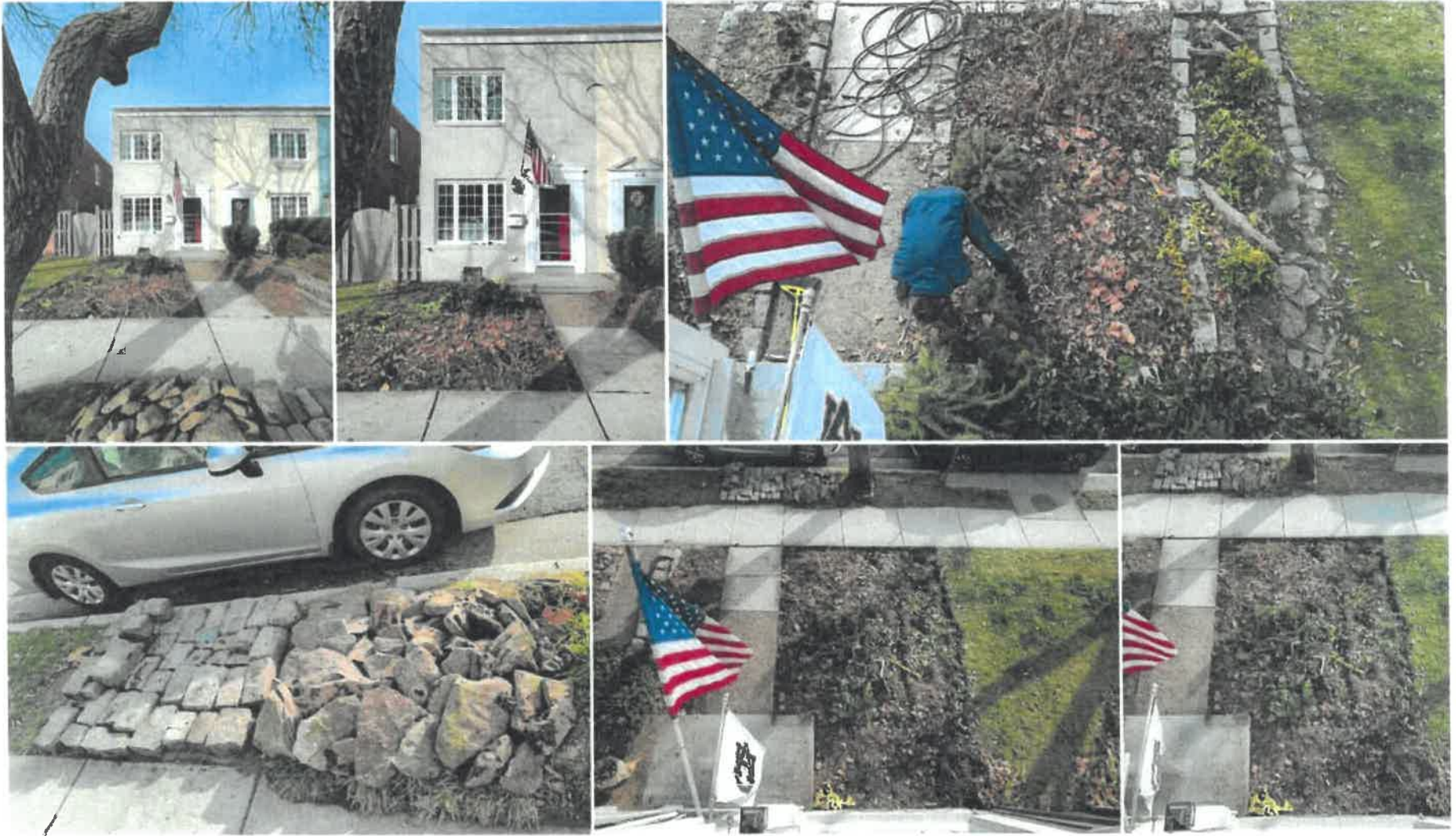
Day 2 Feb 9: Sidewalk and concrete step demolition, raised planter beds footing excavation
