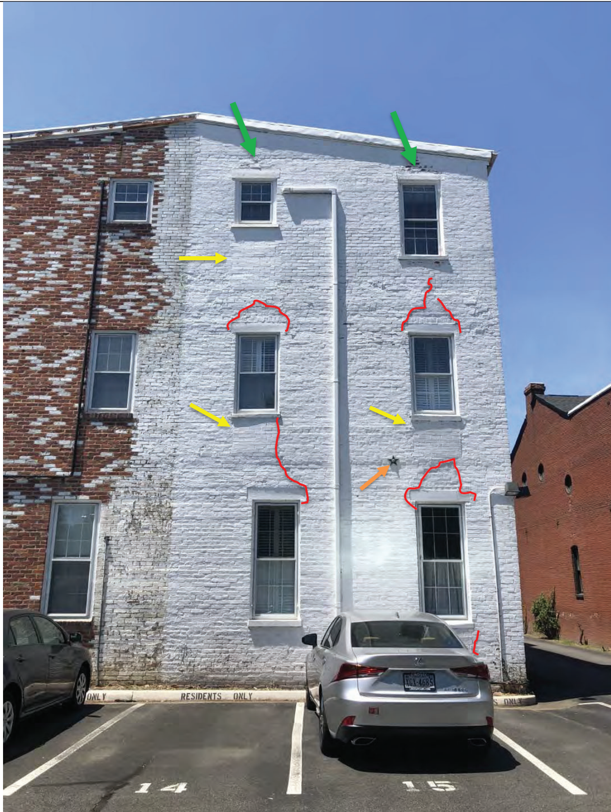
Figure 1: East Elevation with Structural Conditions Noted
