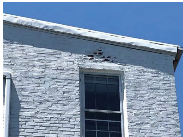
Photo 4: Brick deterioration over lintels
