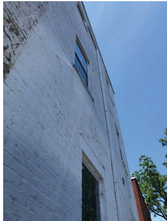
Photo 7: Outward Bowing of East Wall
