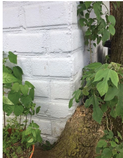
North West Corner of Existing Garage Showing Mitered Textured CMU at the NW Corner.
