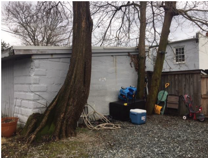
North West Corner of Existing Garage Showing Mitered Textured CMU at the NW Corner.
