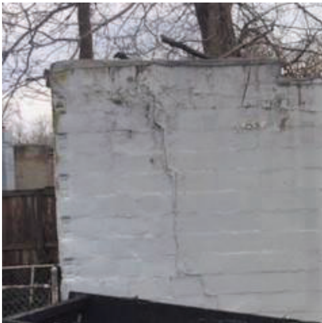
Close Up of South East Corner of Garage; Exposing the “BUTT ENDS” of the Textured CMU Block with Faces South as it transitions to nontextured on the Eastern Wall Face.
