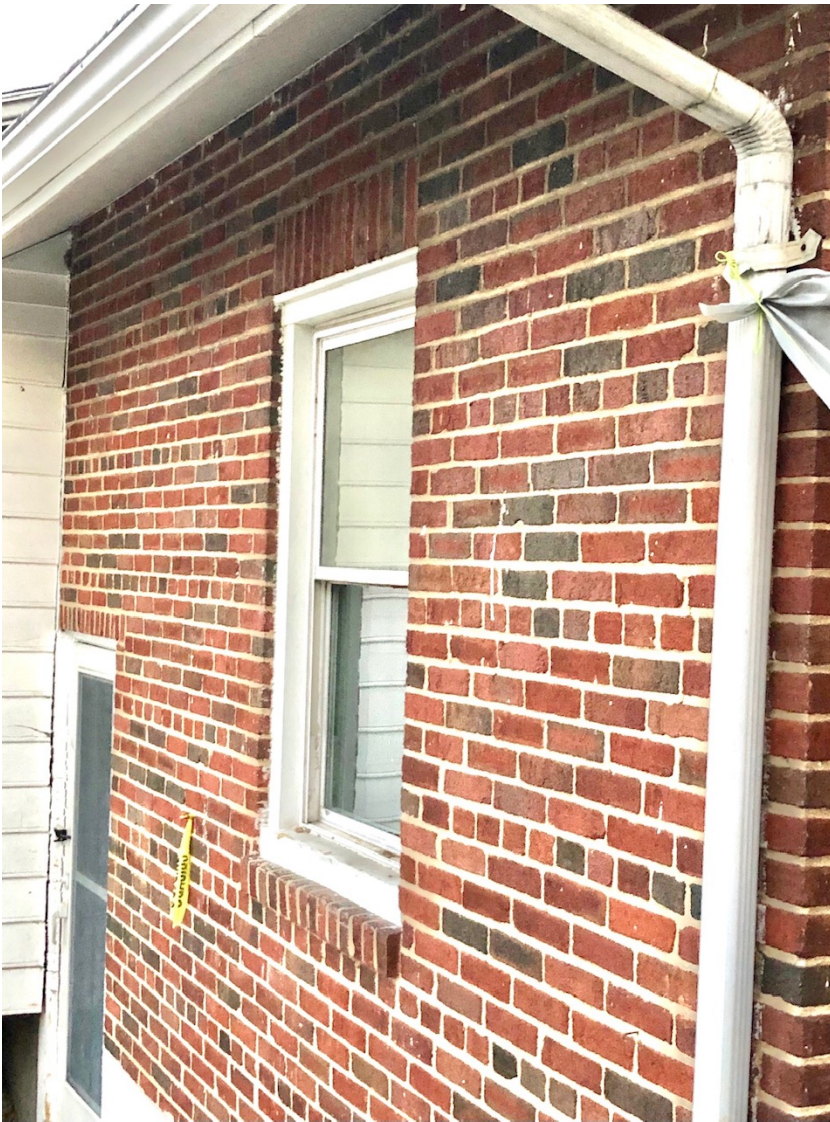
Figure E: Existing bungalow brick details shows - soldier header course or jack arch above window, brick sills and common bond brick pattern with 6 th course headers (every 6 th course) at 7 West Walnut (Existing Bungalow)
