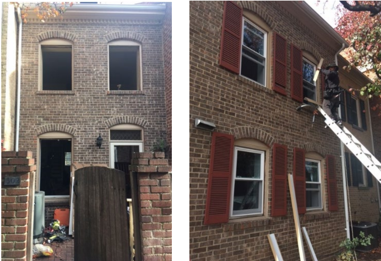
Figure 2: Photographs showing installation of vinyl windows
