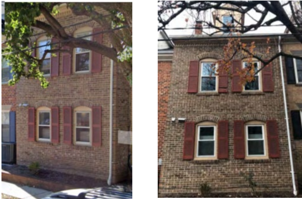
Figure 3: East elevation of property before (left) and after (right) window replacement
