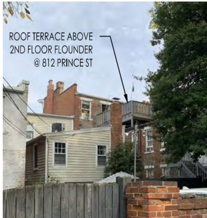
Figure 3: Roof deck at adjacent property
