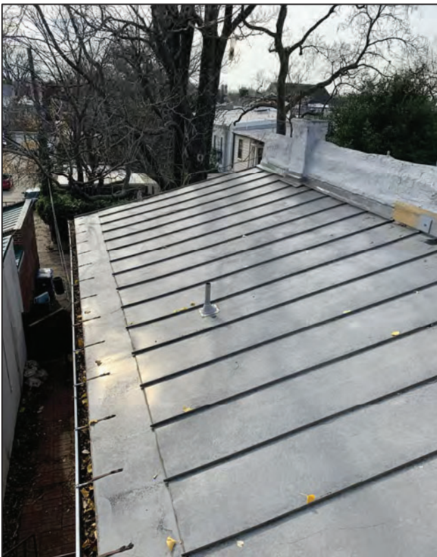
VIEW OF LOW ROOF LOOKING SOUTH
