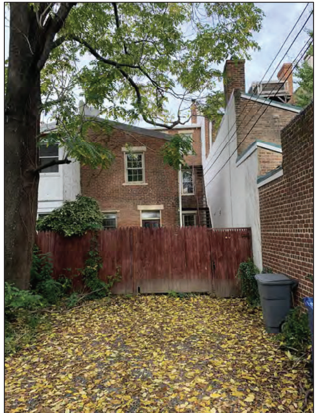
VIEW OF REAR OF FACADE FROM ALLEY
