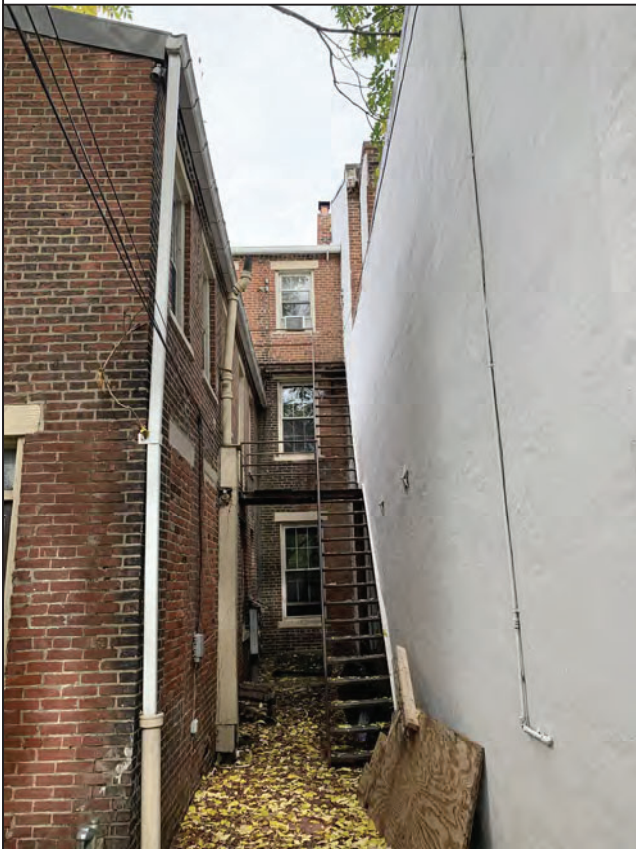
VIEW OF FIRE EXISTING FIRE ESCAPE TO REMAIN
