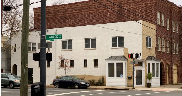
Photo 2: 1000 Queen St. with unapproved paint.
