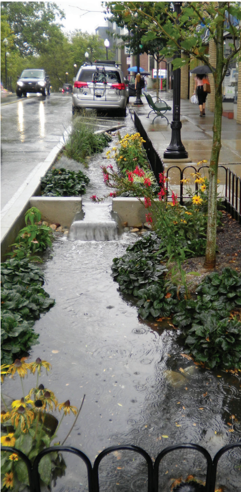
Figure 34. Tree well bioretention basins
