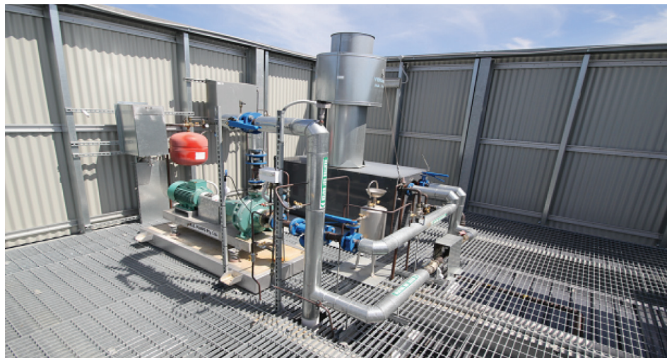
Figure 52. Central domestic hot water
