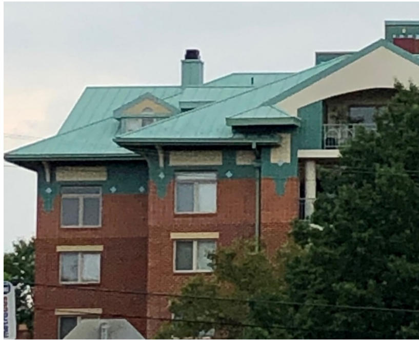
Figure 1: Colecroft Station metal chimneys
