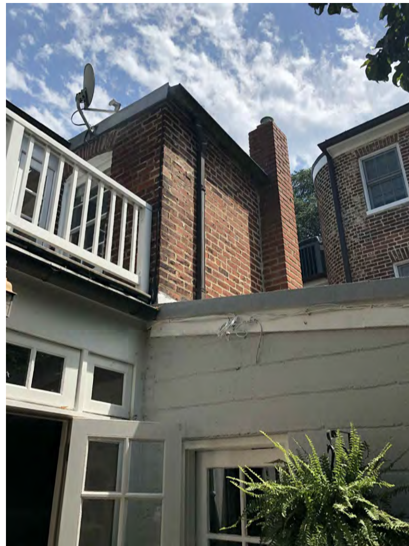
8 REAR EXTERIOR OF 109 S. LEE STREET FACING EXISTING 1 STORY CMU BUMP OUT. EXISTING ROOF TO BE REMOVED, WALLS RAISED 12" AND NEW STANDING SEAM ROOF. NEW WINDOW AT NEW BATHROOM ON SECOND FLOOR
