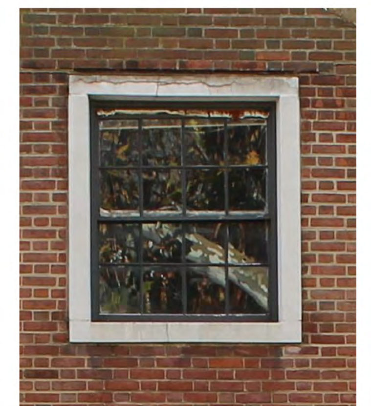
EXISTING CASINGS ARE CRACKED AND FAILING
