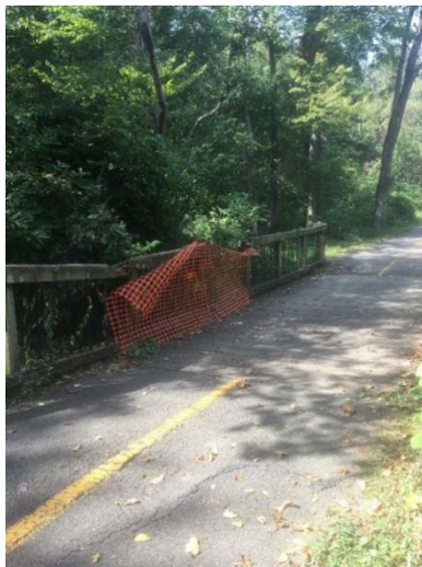
Figure 26: Bridge 2, which needs replacement railings
