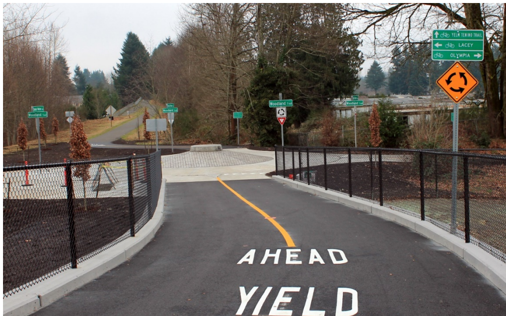
Figure 55: A raised center roundabout at the intersection of the Woodland Trail and Chehalis-Western Trail in Olympia, Washington (Source: Jonah Finkelstein, Mike on Traffic)
