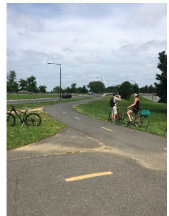
Figure 17: Example of trail cracking and weed encroachment
