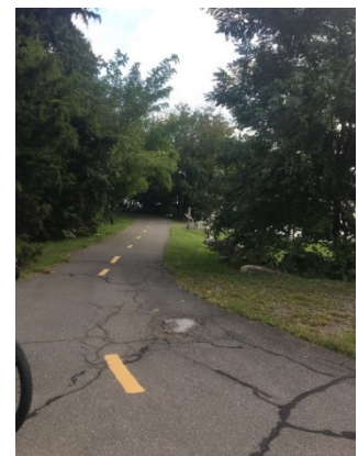
Figure 18: Example of trail cracking and uneven surface
