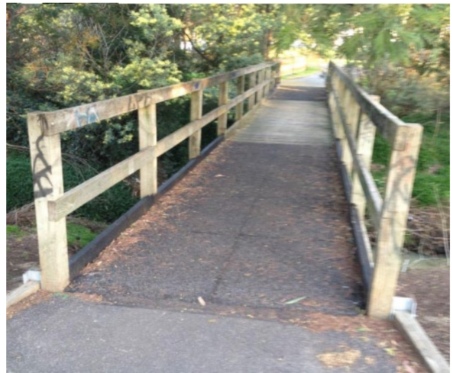
Figure 46: A timber bridge with asphalt patch (Source: Downer EDI)
