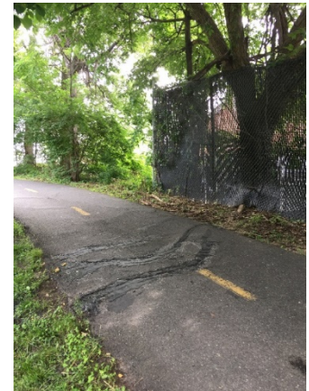
Figure 16: Example of pavement ruts
