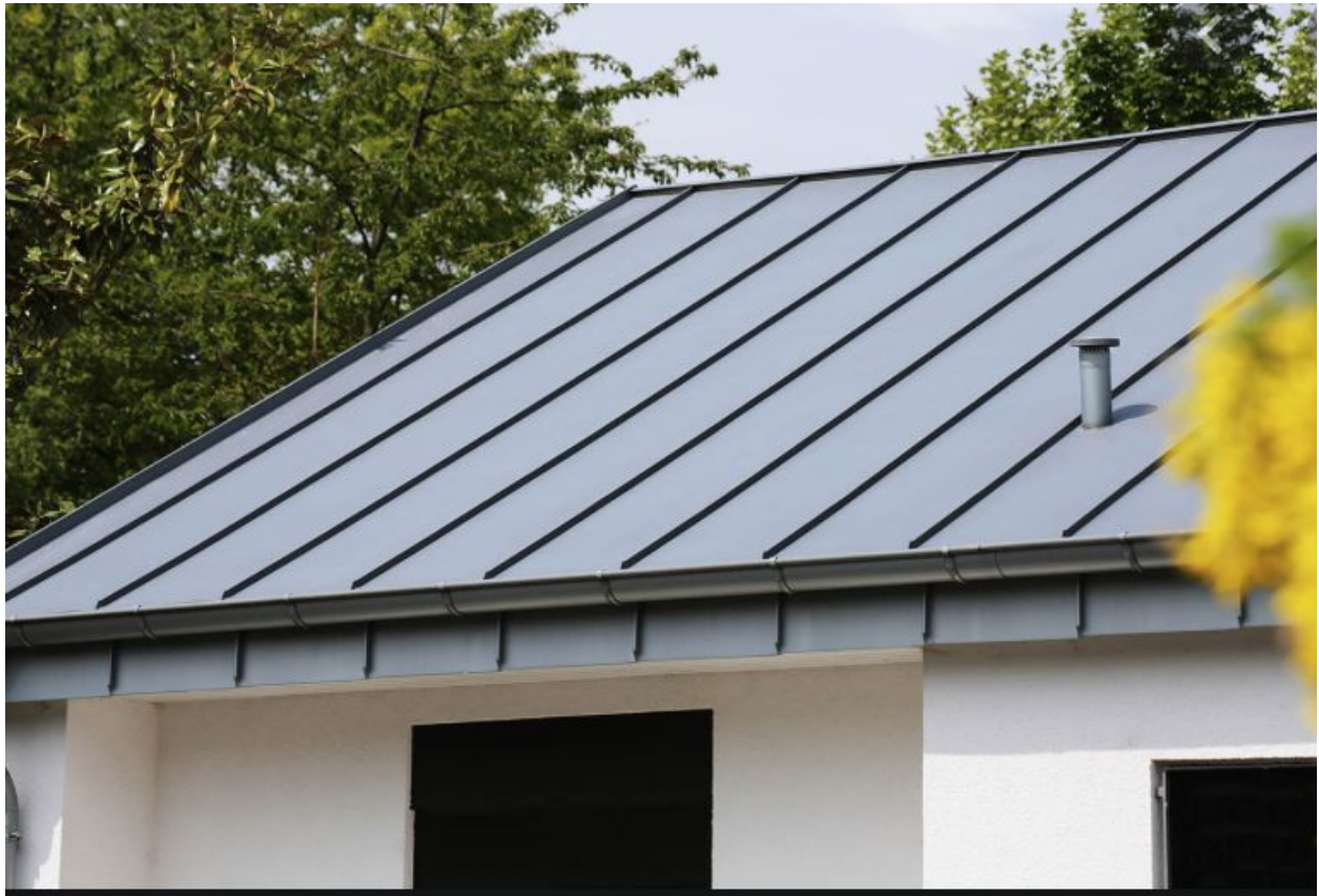
Roof- Black Standing Seam Metal
