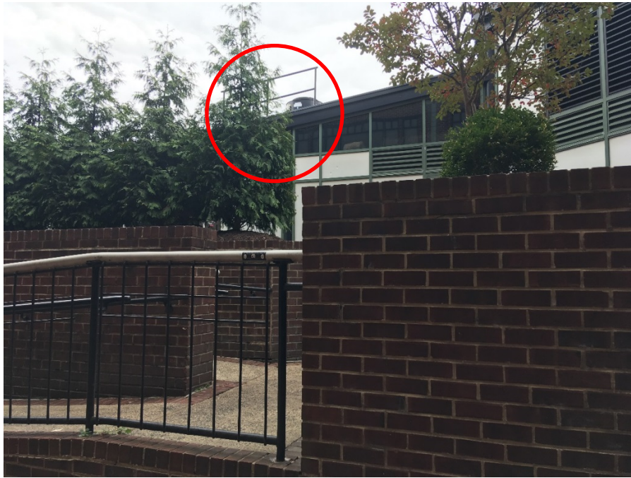
Figure 2 – Guardrail to be revised at existing kitchen exhaust vents
