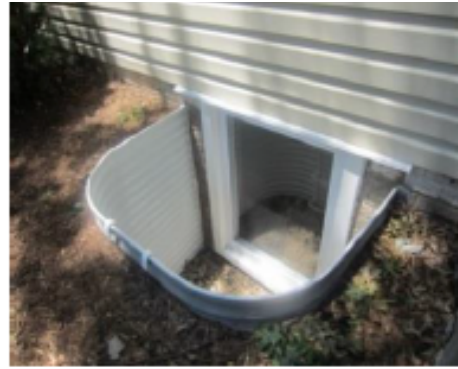
Figure 11: Neighboring property with identical Bowman Kemp Easy well with window, metal grate and plastic cover, installed in the same manner as this proposal.
