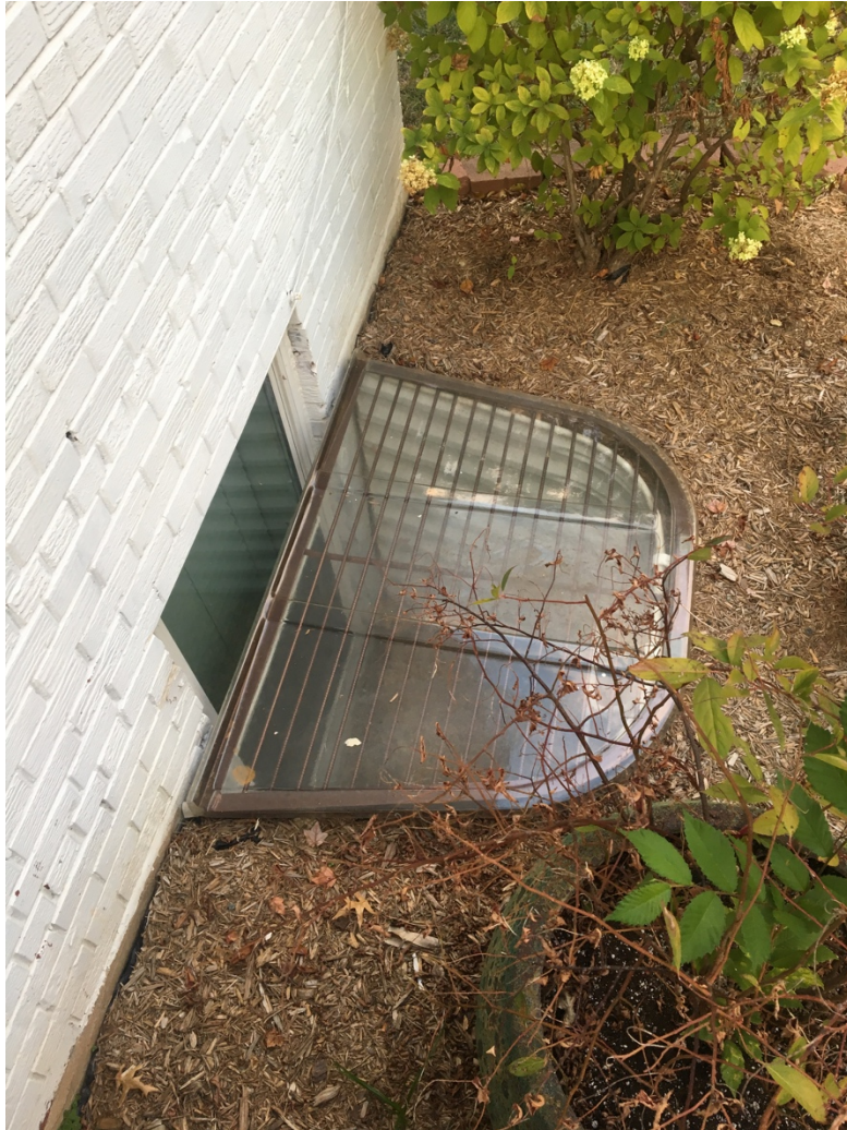
Figure 12: Neighboring property with identical Bowman Kemp Easy well with window, metal grate and plastic cover installed in the same manner as this proposal.
