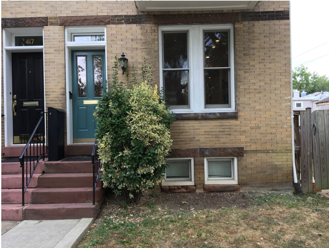
Figure 1: Photo showing existing front façade with two basement windows (27 ¼" x 22")
