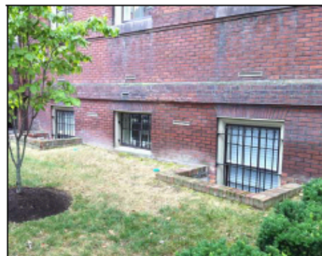
The windows on this school building have been lowered within new window wells that are unobtrusive to the building and site.
