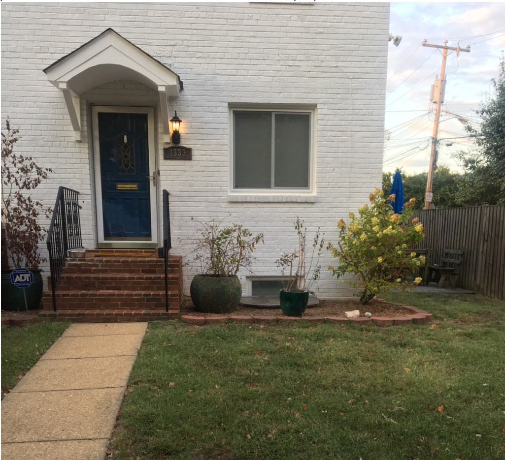
Figure 11: Neighboring property with identical Bowman Kemp Easy well with window, metal grate and plastic cover, installed in the same manner as this proposal.
