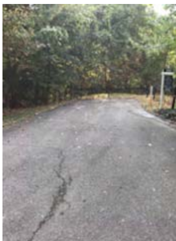
Sample Roughness/Cracks in Paving
