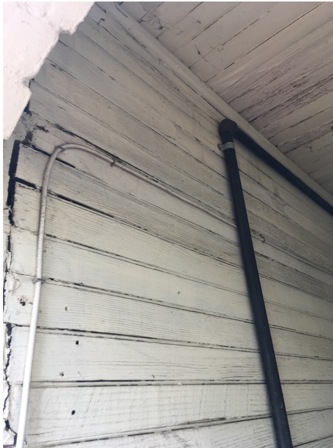
Figure 3: Beaded siding on the west wall of the horse alley
