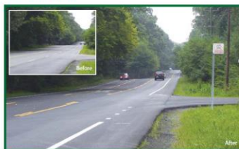
Lawry's Road, before and after a 2009 Road Diet Source: Randy Dittbemer, Virginia DOT
