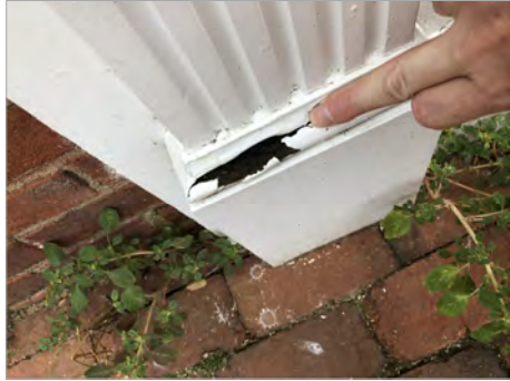
WATER DAMAGE - REPLACE OR PATCH DAMAGED WOOD TRIM
