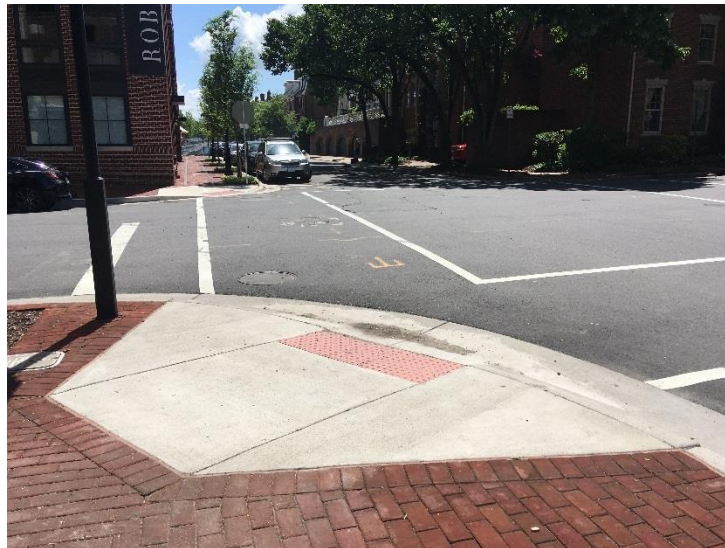
Figure 2: New concrete curb ramps in brick sidewalks at Princess and North Columbus streets
