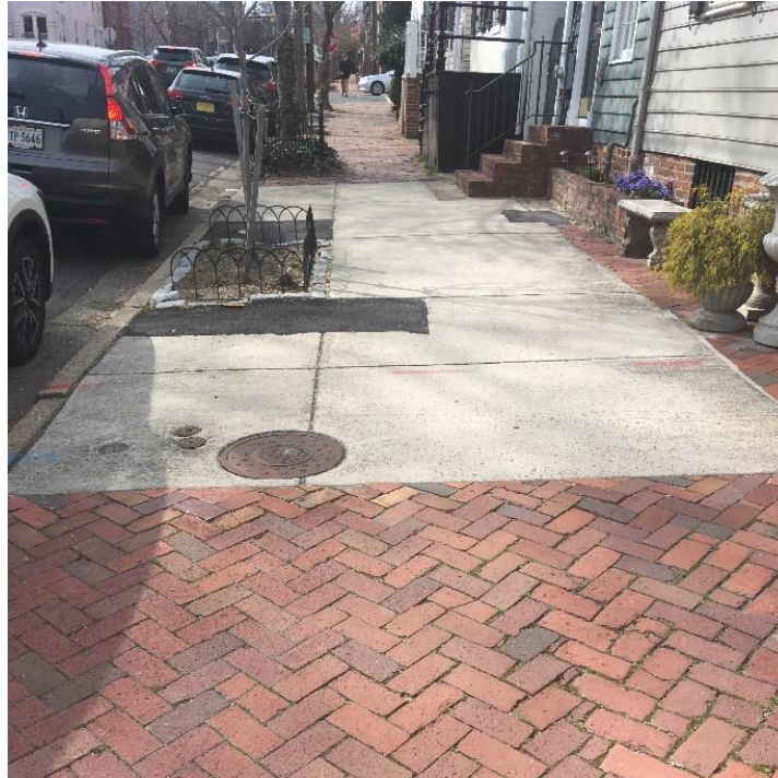
Figure 1: Queen Street brick sidewalk with concrete section
