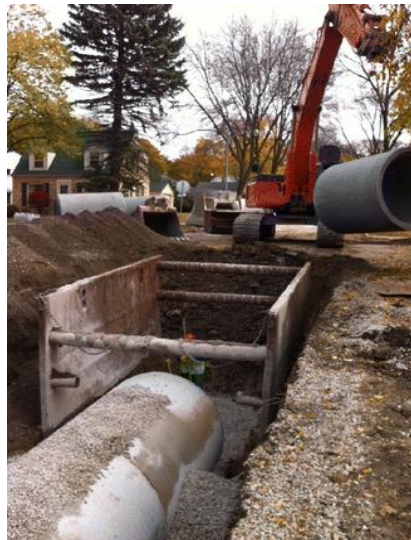
Hooffs Run Tunnel (open-cut)
