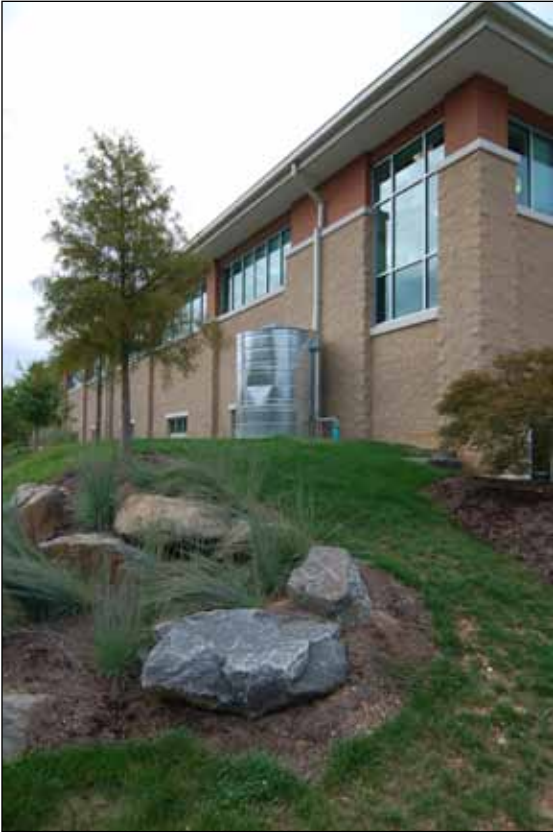
Figure 8-5. Cisterns For Greywater Re-use, Arlington, VA
