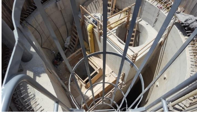
Shaft internal concrete (upper shaft)
