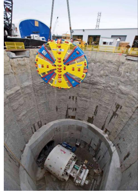
Finished shaft excavation support
