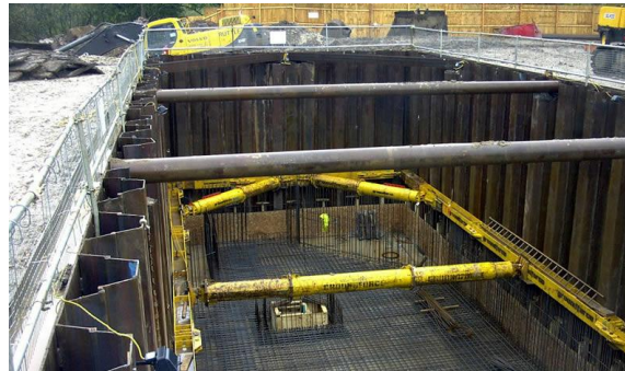
Braced sheet pile wall
