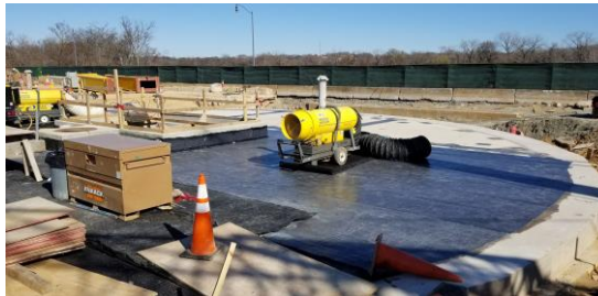
Shaft cover and backfill
