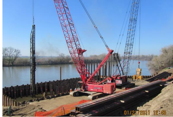
Work within sheet pile wall
