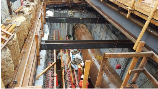
Excavation support and flume
