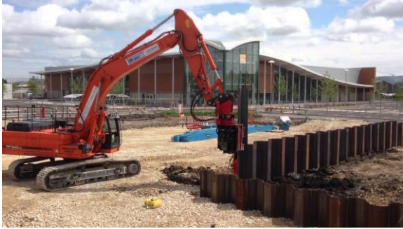
Sheet pile installation
