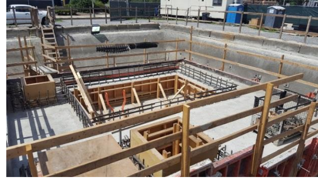
Concrete formwork and pours
