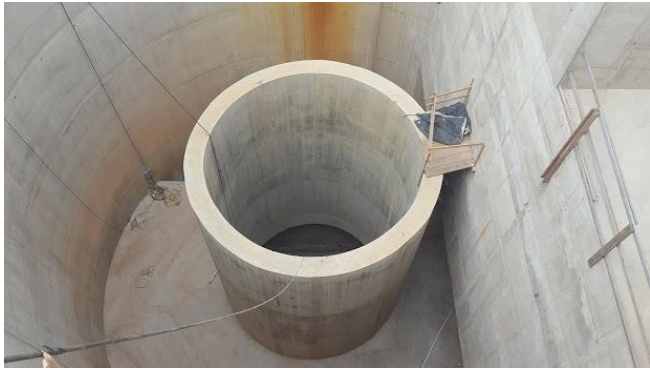
Shaft internal concrete (lower shaft)
