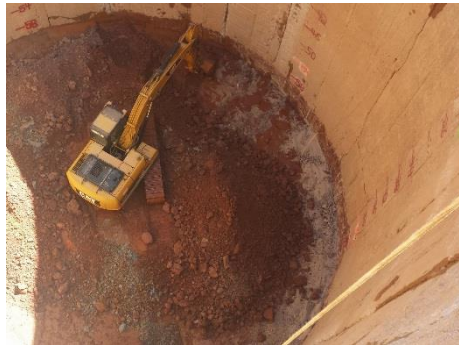
Shaft excavation
