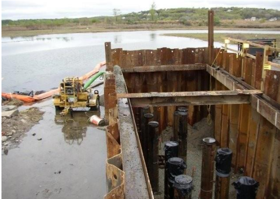
Finished sheet pile wall
