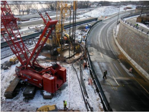
Shaft excavation support installation
