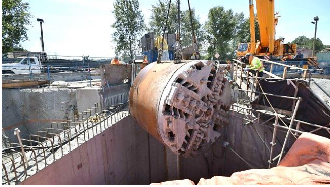
TBM removal
