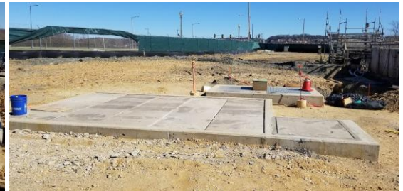
Shaft cover and backfill
