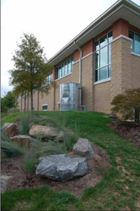
Figure 8-5. Cistems For Greywater Re-use, Arlington, VA
