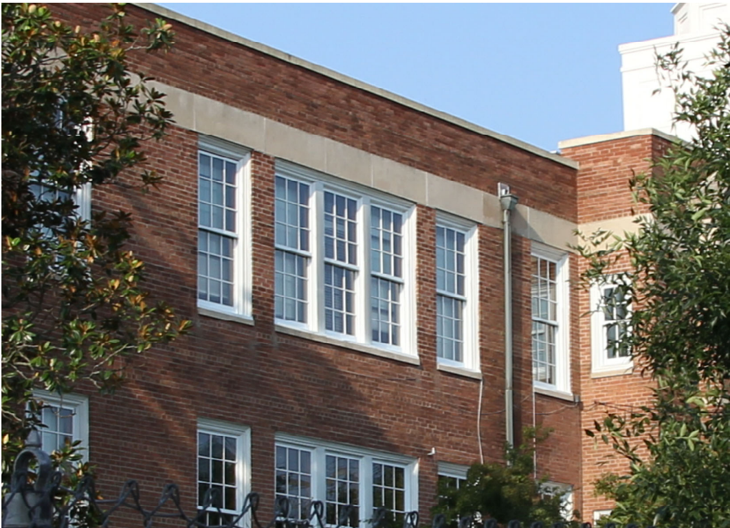
NORTH FACADE OF MAIN BUILDING: SHOWING TYPICAL BRICK WALL; STONE COPINGS, BELT COURSES, AND SILLS, AND ALUMINUM CLAD WINDOWS
