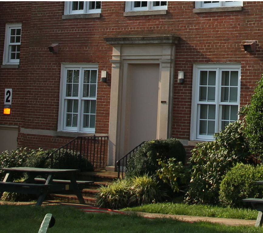
SOUTH FACADE OF STEPHENS HALL: SHOWING TYPICAL BRICK, STONE ARCHITECTURAL TRIM AND WINDOW SILLS, STONE COPINGS, PAINTED METAL RAILINGS
