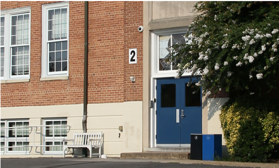
EAST FACADE OF MAIN BUILDING: SHOWING TYPICAL BRICK AND PARGED/PAINTED CONCRETE BASE
