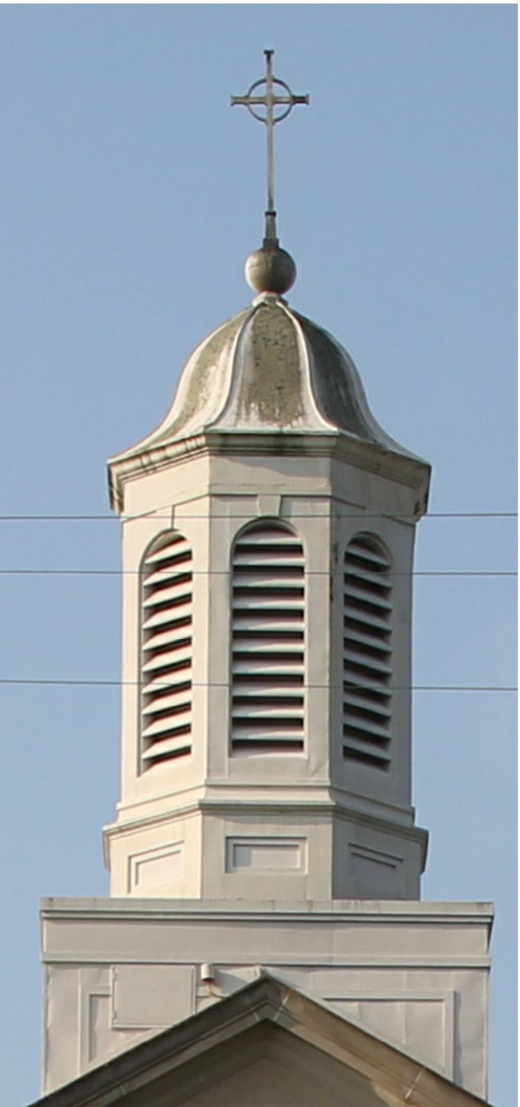
CUPOLA OF MAIN BUILDING: SHOWING METAL ROOFING MATERIAL
