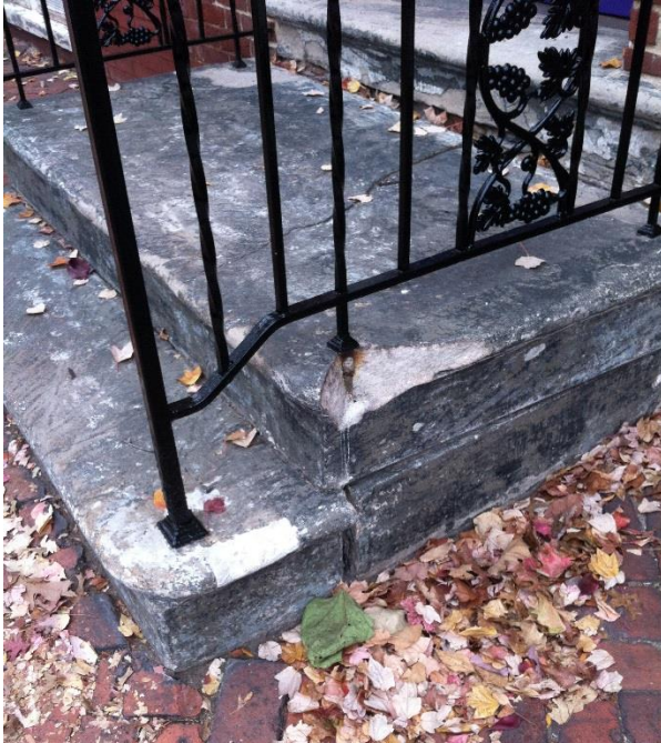
Photo 9: Damage to stone steps from rusting iron railing
