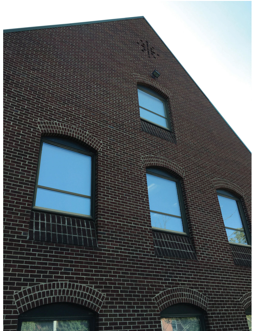
PHOTO 2 - PROPOSED WINDOW REPLACEMENT WITH DARK BRONZE AND ANODIZED ALUMINUM FRAME WITH AWNING UNIT ON BOTTOM PORTION
