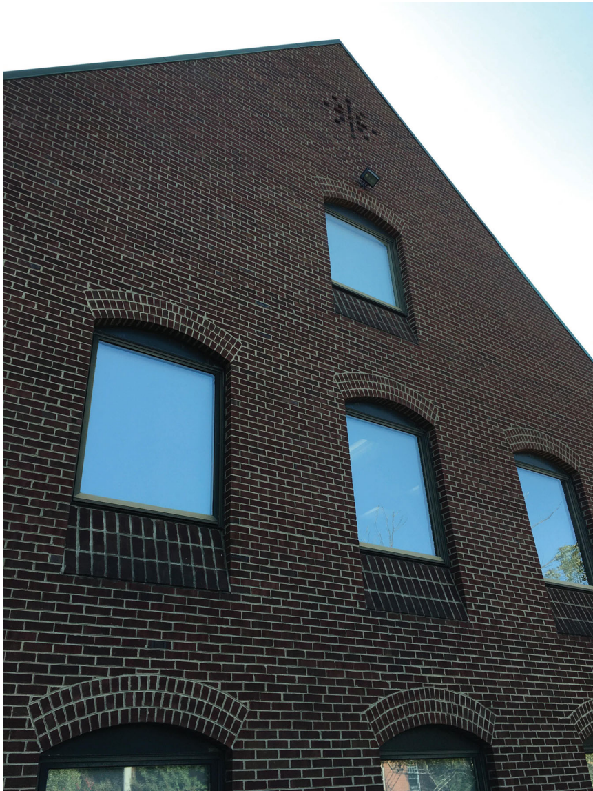
PHOTO 1 - EXISTING WINDOWS - SINGLE FIXED UNIT WITH BRONZE ANODIZED FRAME AND TINTED GLASS
