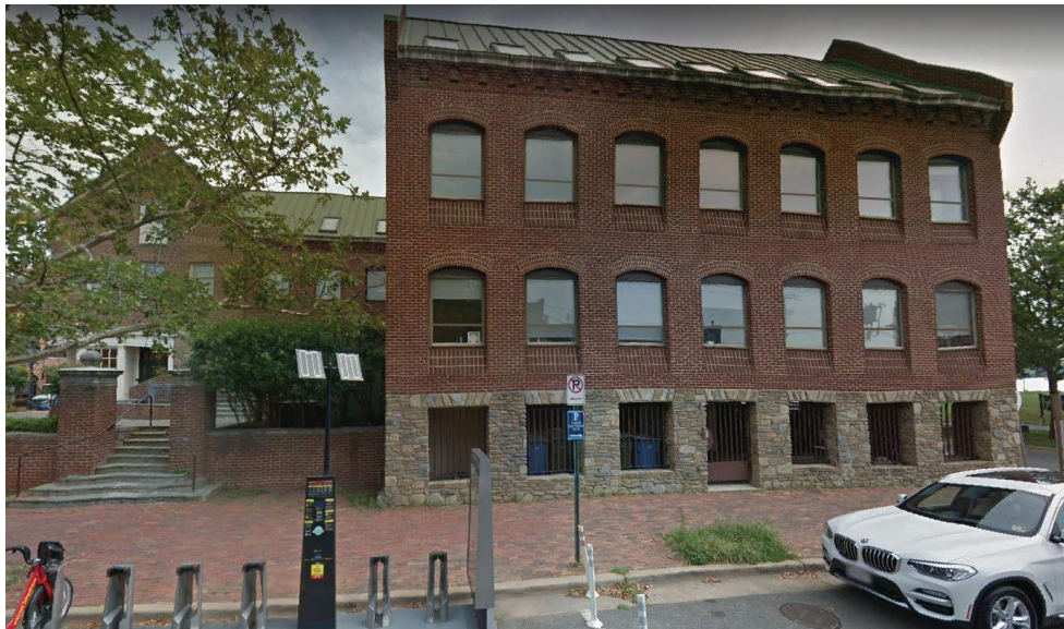
PHOTO 2 - PROPOSED WINDOW REPLACEMENT - SINGLE FIXED UNIT ABOVE AWNING UNIT WITH BRONZE ANODIZED FRAME AND INKIND REPLACEMENT GLASS
