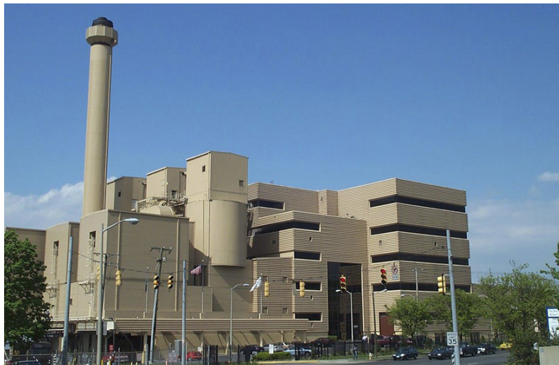
Figure 14 Covanta A/A Waste-to-Energy Facility
