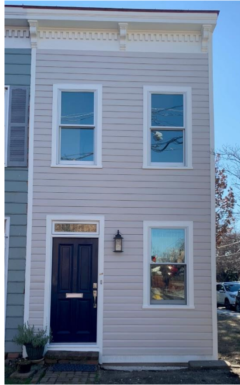
Figure 3: Current Franklin Street elevation showing historic German siding, painted wood door and aluminum-clad windows.
