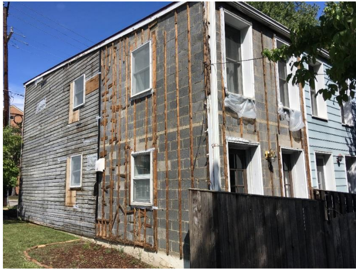
Figure 1: View looking northeast taken by staff on August 31, 2018 showing the CMU rear addition to the original structure.
