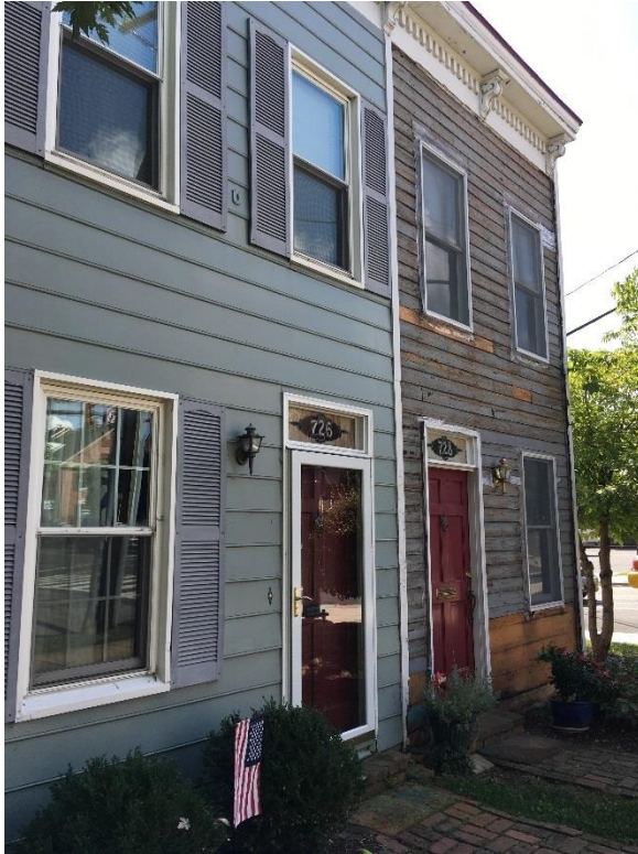
Figure 2: Front façade after removal of Masonite siding.
