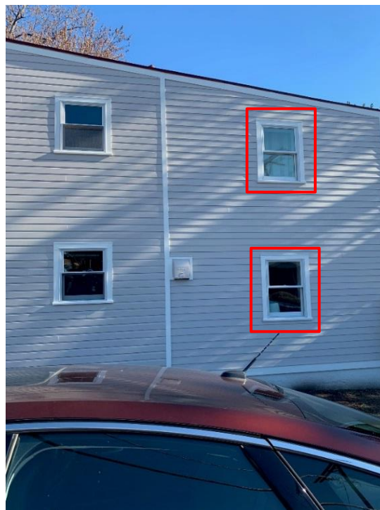
Figure 4: Existing aluminum-clad windows on the South Columbus Street elevation. The two outlined windows are located on the 1978 addition and comply with the BAR's window policy.
