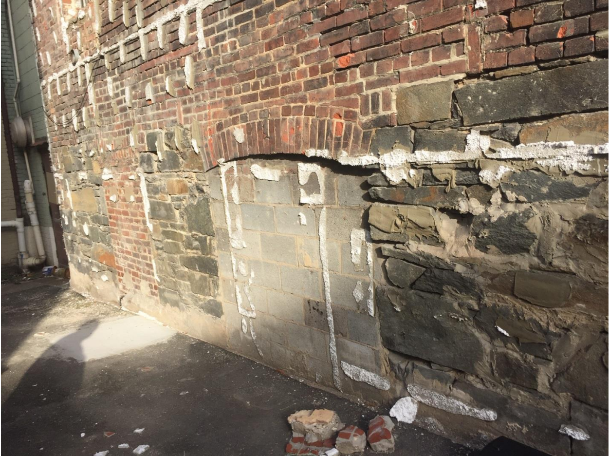
Figure 1. West elevation showing remaining stone foundation and damaged brick above. The cement can be removed from the stone with limited damage however extensive damage occurs to the brick when it is removed.
