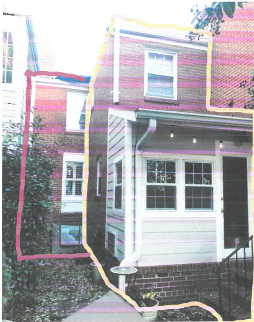
515 S Fairfax – Rear elevation of structure to be demolished. Area to demolish is in yellow. Area to encapsulate is in red. Additional photographs are provided with the drawings.
