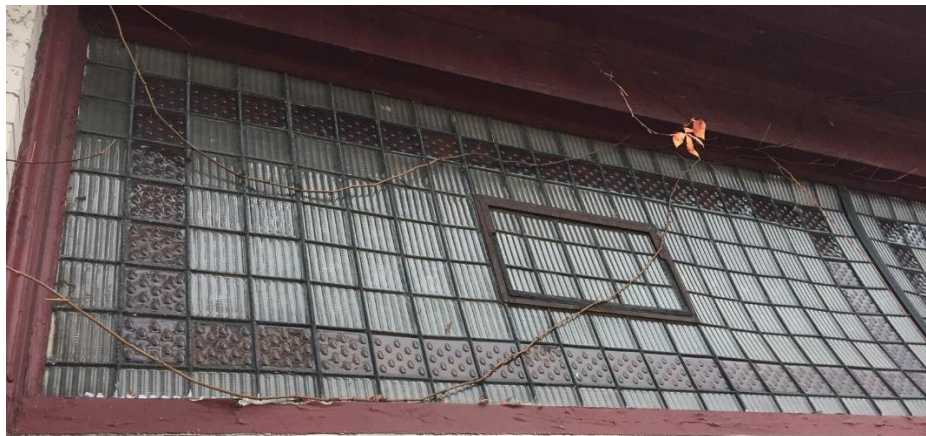
Figure 1. Existing pressed glass transom at 1320 Prince Street.
