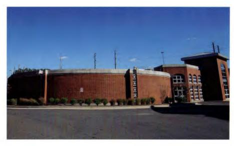
Our digesters are the home of microbes that break down organic matter in the water and produce gas that we collect and use as energy.
