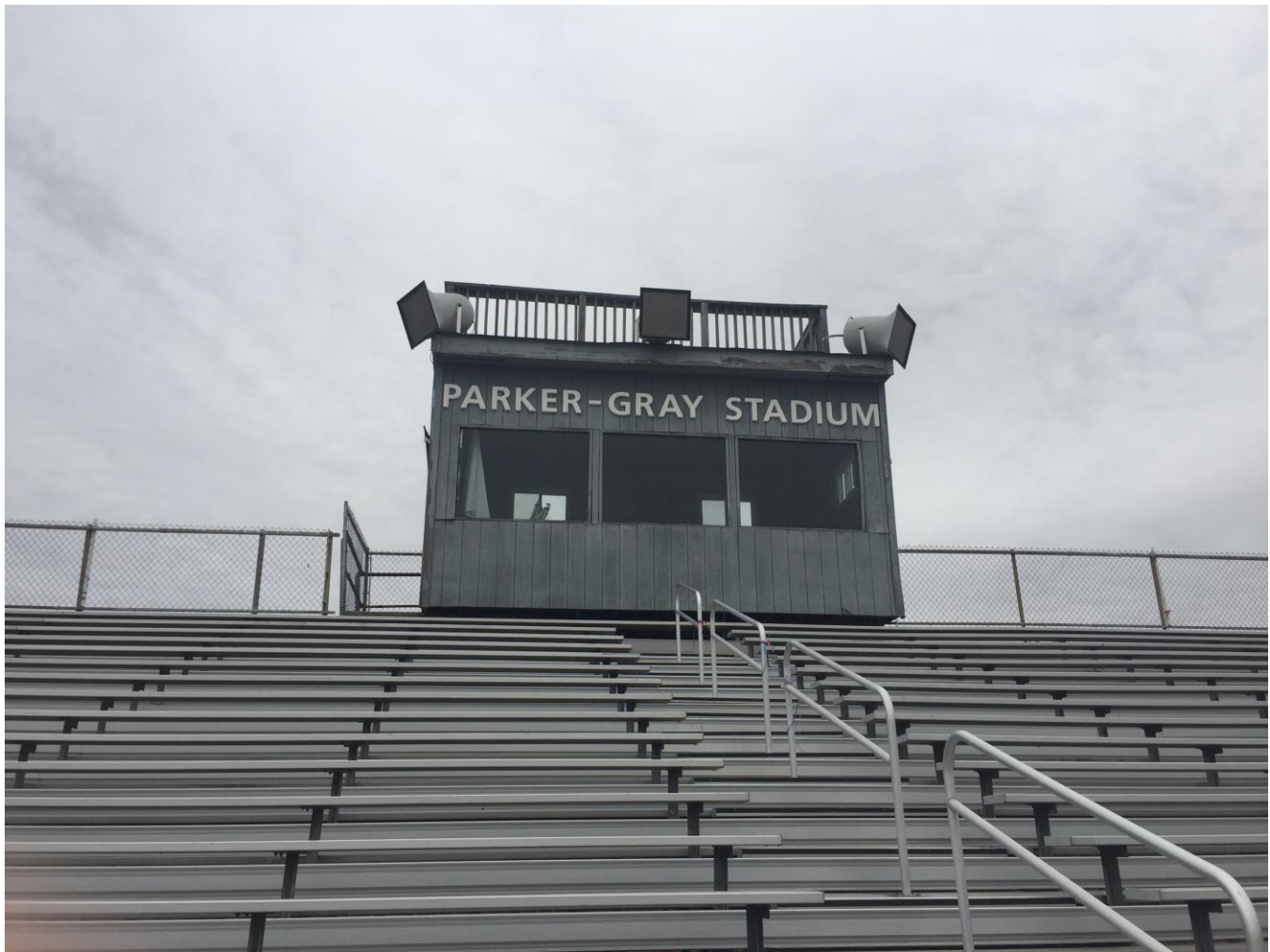
Image 1: Existing Press Box and loudspeakers at ‘Home’ bleachers. Note poor aiming of the loudspeakers
