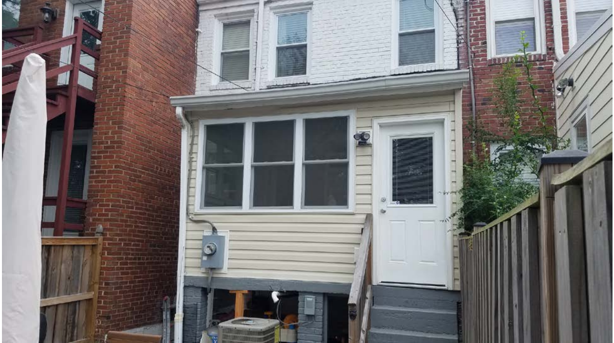
Photograph of rear enclosed porch/sunroom to be demolished. Wooden brace in center is currently aiding in support of deteriorating masonry/cracking of concrete supports.
