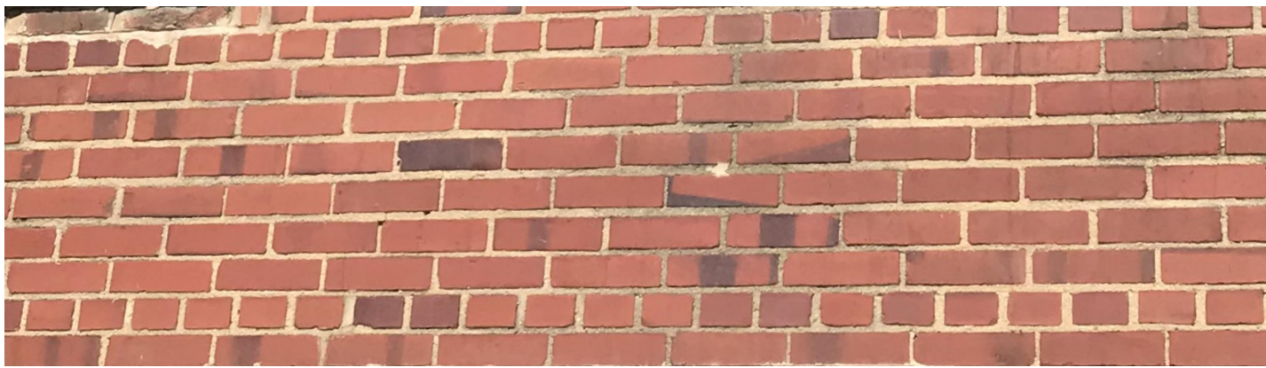
EXISTING BRICK W/ NEW BRICK TO MATCH
