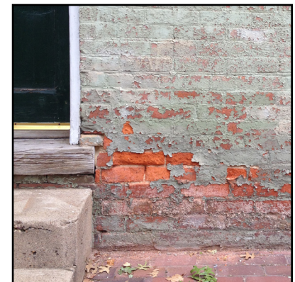
Rising damp (water wicking from below) has caused the face of this early brick to crumble from the freeze-thaw cycle.
