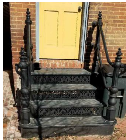
Figure 4- Proposed steps and railings will match the cast iron stoop at 1301 Prince St.
