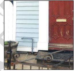
Meter must remain in the basement but a pressure relief valve may be located on the front or side façade. Paint valve and pipe to match adjacent wall color.
