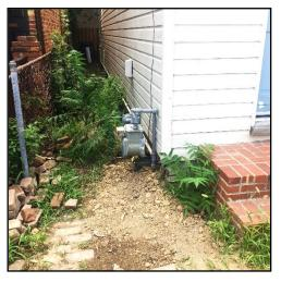
Meter may be located in the side yard behind the façade. Paint meter to match adjacent wall color and screen with landscaping or fence.
