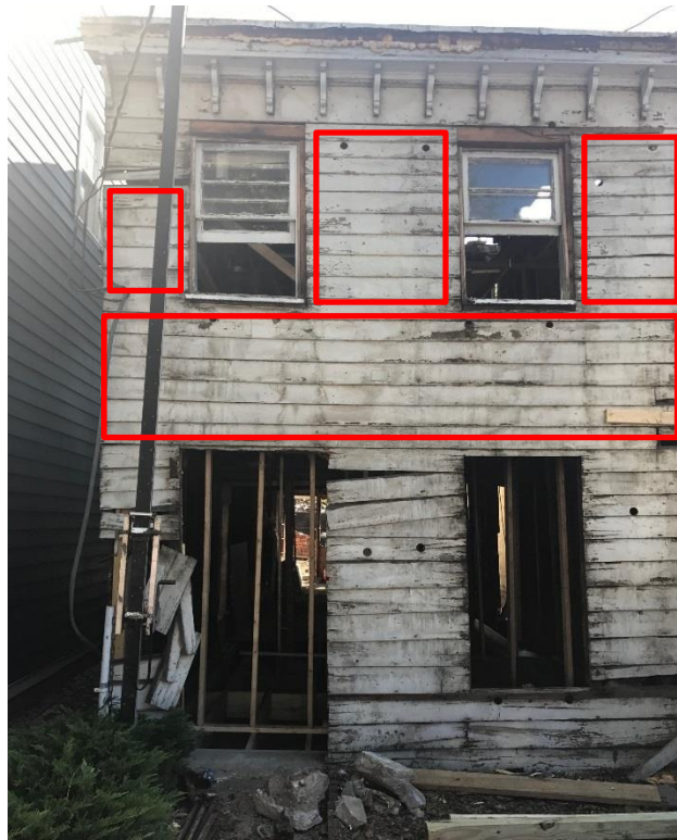
Figure 1: Historic wood siding on front (west) elevation. Red rectangles indicate areas containing significant proportions of siding material that staff determined should be repaired and retained.
