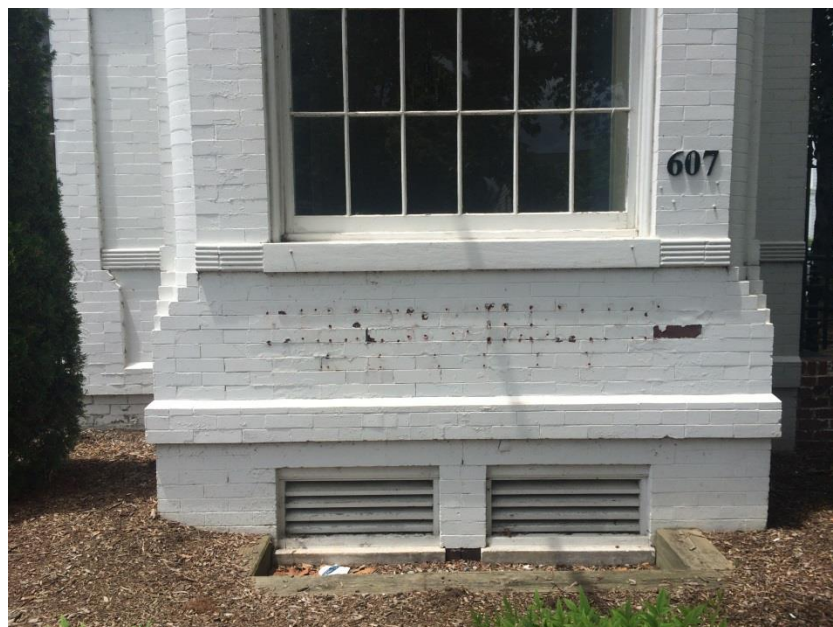
Figure 2: masonry damage caused by pin mounted signs
