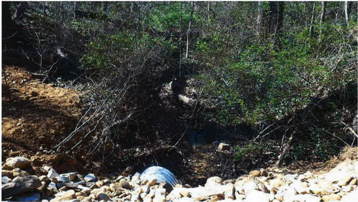
Fig. 7. Upstream intake of spring-fed, mostly perennial stream into galvanized pipe underlying an area at 2208 Russell Road where the stream was filed in with massive amounts of soil. Photo by R.H. Simmons.
