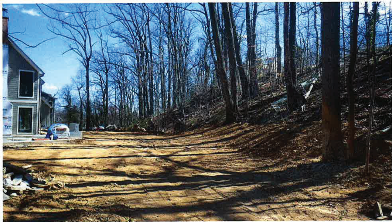
Fig. 6. Middle section of filled in stream channel at 2208 Russell Road showing damaged trees and buried toe and lower slope of old-age forested ravine. Photo by R.H. Simmons.
