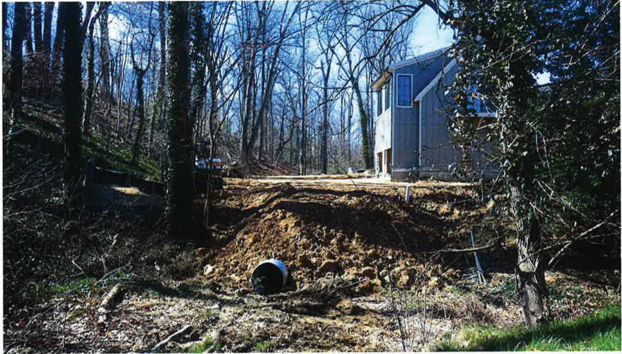
Fig. 5. Large-scale filling in of the mostly perennial, natural-channel, spring-fed stream at 2208 Russell Road. Pictured here is the outflow of the galvanized pipe that spans the filled segment – a considerable stretch of the ravine. Photo by R.H. Simmons.
