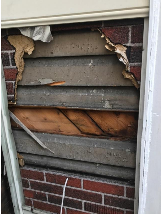
Figure 1: Exposed German lap siding on ell
