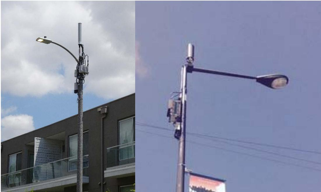
*Figures 1, 2: Typical Small Cell Facility installations*
