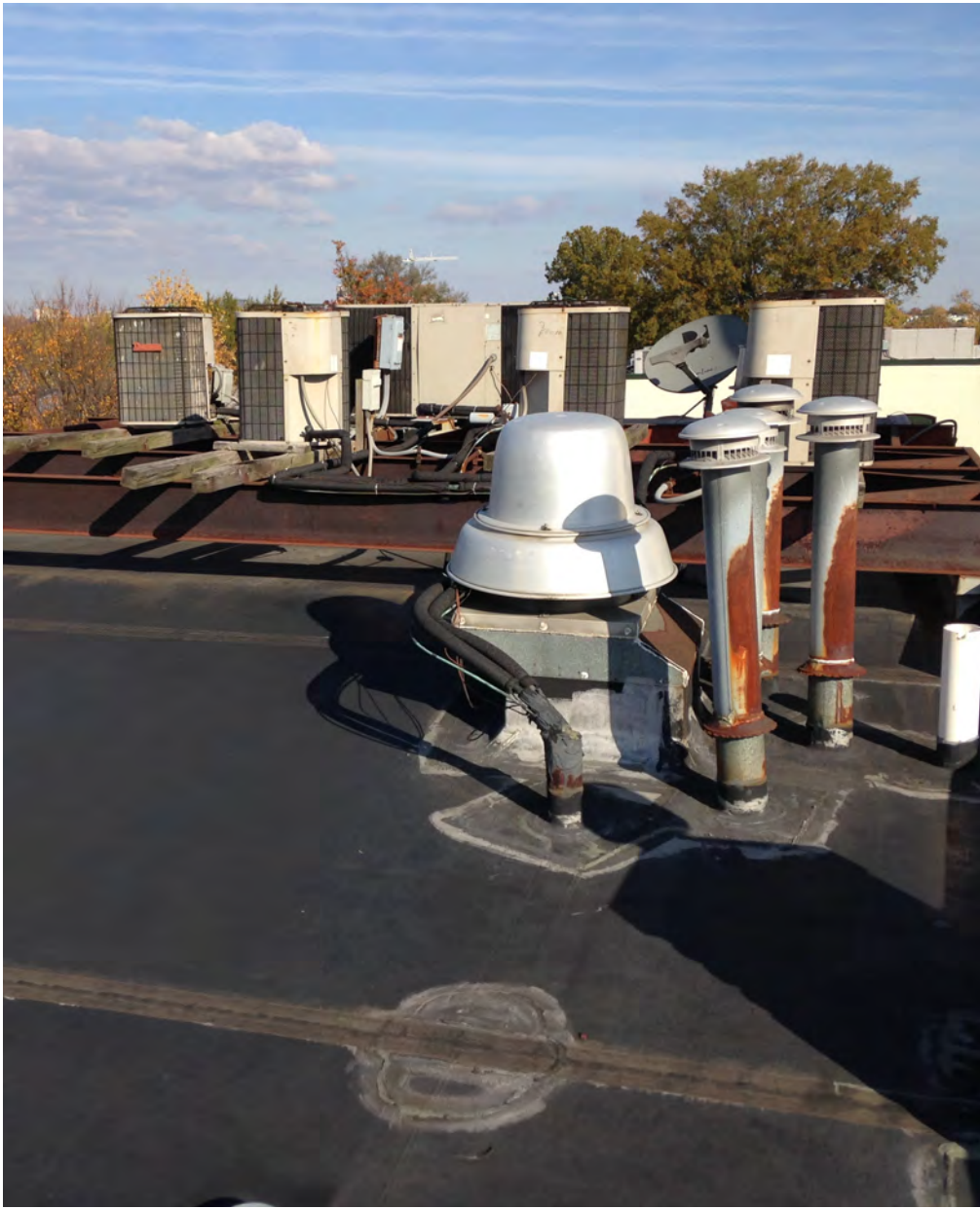
EXISTING ROOF DUNNAGE AND EQUIPMENT
