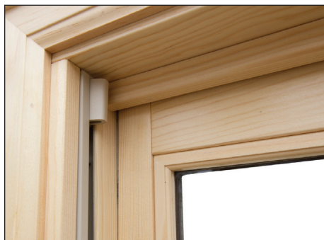
Wood Parting Stop, Concealed Jambliner
